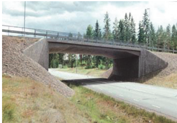
Figure 1. A concrete slab frame bridge [18]
