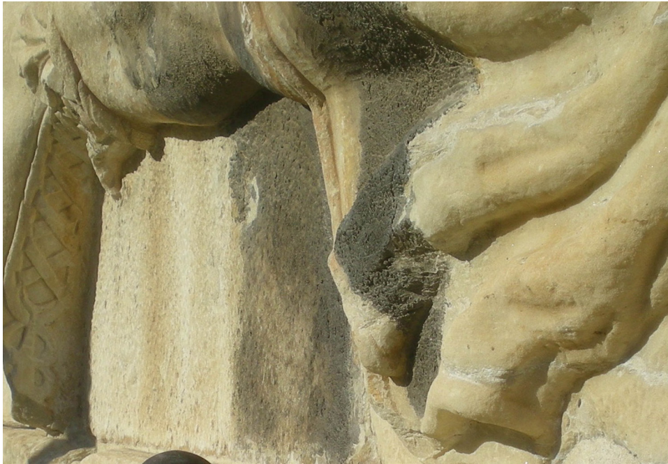
Fig. 2 Black crusts on the Tower's frieze, Tower of the Winds (photo credit: Greek Ministry of Culture & Sports - Fund of the Archaeological Proceeds)
