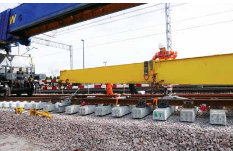
Fig. 6. Integrated turnout installation process at Psary Station Source: own archive.
