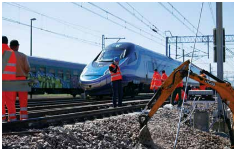
Fig. 4. Process of the turnout installation
