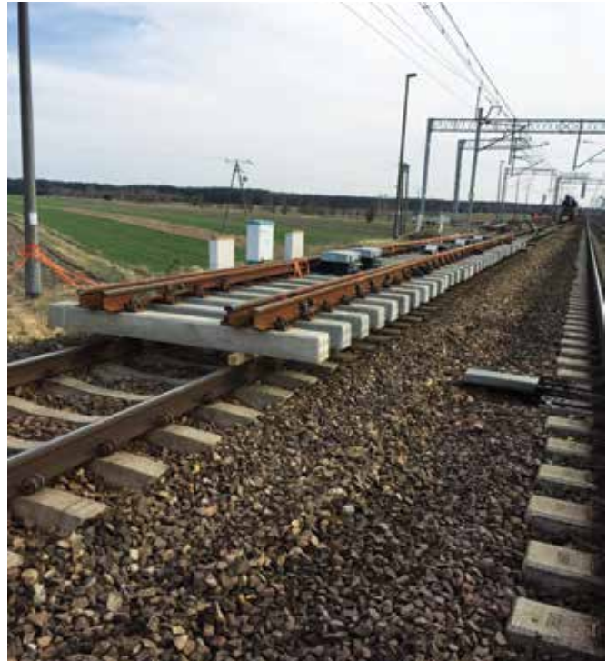
Fig. 3. Switch panel prepared for installation
