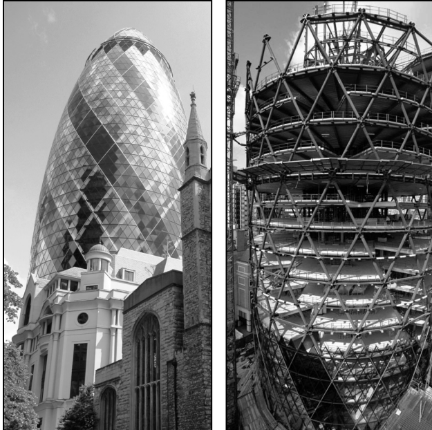
Figure 1: 30 St. Mary Axe Tower, London: a view – the form and the steel structure under construction source: K. Foljanty and www.constructalia.com/repository/transfer/en/resources/ContenidoProyect/00919849Foto_big.pdf
