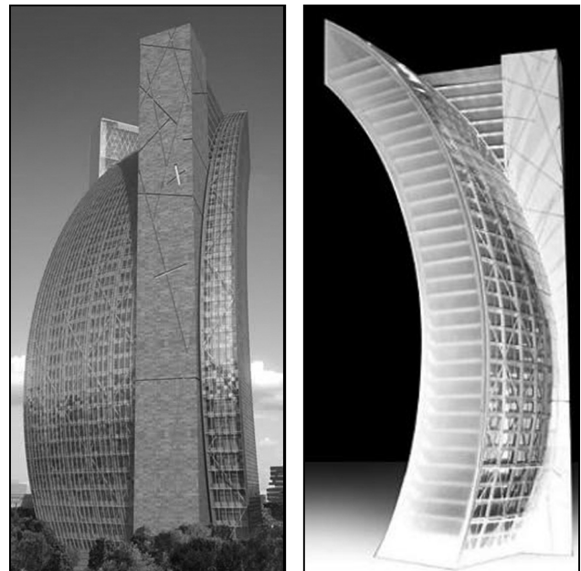
Figure 6. Il Curvo Tower, Milan: a visualization – the form and a model of the structure. source: saint-andres.blogspot.com/2010/06/milano-progetto-city-life-3-grattacieli.html and www.idealista.it/news/immobiliare/residenziale/2010/05/19/6292-ti-piacerebbe-vivere-in-un-grattacielo
