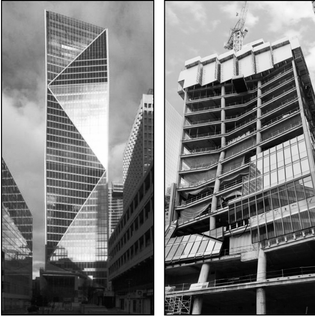
Figure 3. Carpe Diem Tower, Courbevoie: a view – the form and the reinforced concrete structure under construction. source: www.ramsa.com/en/news/tour-carpe-diem-certified-lead-platinum-raising-ramsa-s-total-to.html and www.doka.com/web/newsroom/press/Tour-Carpe-Diem.me.php
