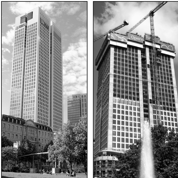
Figure 2. Opernturm, Frankfurt: a view – the form and the reinforced concrete structure under construction. source: commons.wikimedia.org/wiki/File:Frankfurt Opernturm_(Taunus anlage).jpg and www.skyscrapercity.com/showthread.php?t=1328795&highlight=frankfurt&page=2
