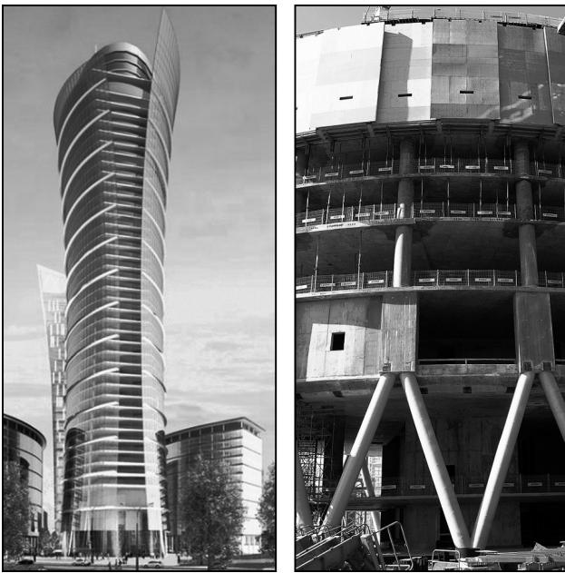
Figure 8. Warsaw Spire, Warsaw: a visualization – the form and the steel and concrete structure under construction. source: www.skyscrapercity.com/showthread.php?t=596467&page=5 and www.cbakkala.com/project/warsaw-spire-poland
