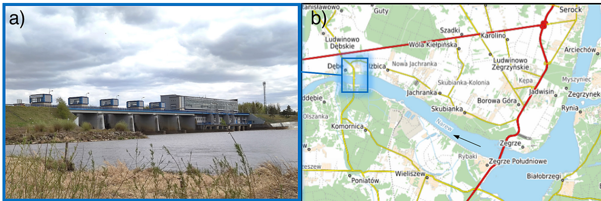
Figure 1. Dębe hydropower plant in Central Poland as an example of run-of-the-river project (Author of photography: Marta Kiraga, 2020); a) the view from downstream location; b) the valley topography
