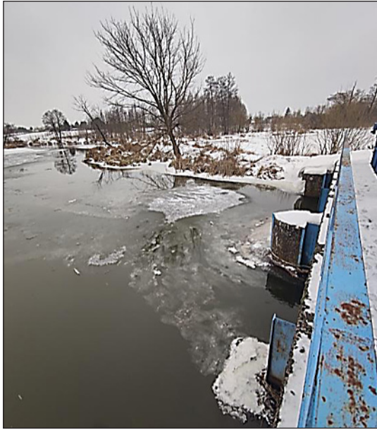
Figure 8. Ice cover retained upstream the hydraulic structure on the weir (Radomka river in Central Poland at river kilometer 44 + 000 – winter 2021, author: Marta Kiraga).
