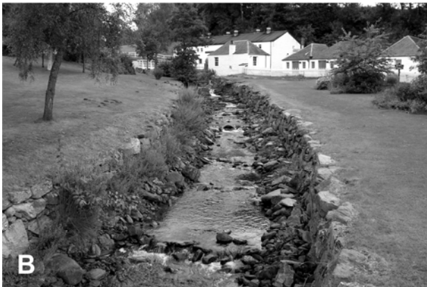
Photo 1. Examples of artificial, stone lined open channels of different scenic attractiveness and environmental impact: (A) artificial channel of Łopuszna Stream, Polish Carpathians, with an impervious, smooth bottom, inhospitable to benthic biota, and with fast water flow precluding the existence of habitats for fishes and their upstream migration to spawning places. (B) artificial channel from Scotland showing a gravelly bed with a sequence of steps and pools, providing habitats for aquatic biota. (photo by B. Wyźga).
