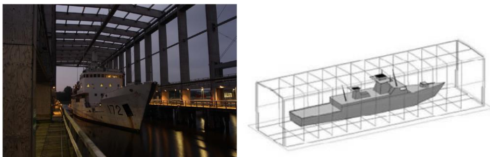
Fig. 4. CFAV Quest inside EFS (left) [1] and schematic drawing of EFS with ship inside (right) [2]
