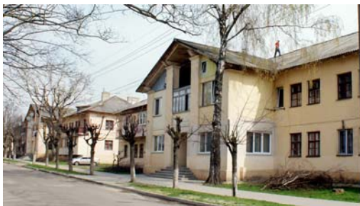
Fig. 12. Residential building (1950-ies), settlement "Zhovtneve" (Levandivka), Source: photo I. Cherniak, 2018
