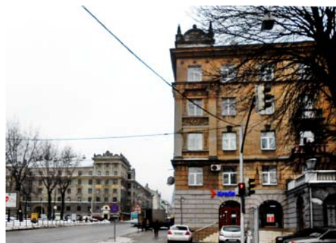
Fig. 15. Residential building on the corner of Gorodotska and Y. Mudryi Streets and another one on Gorodotska - Ozarkewycha St. in the background. Source: photo by I. Cherniak, 2018.
