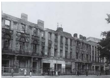
Fig. 18. The destroyed building of the Credit Society at the corner of Lenin Avenue (Svobody Avenue) and Copernicus Street, photo of the 1940s. Source: [8]
