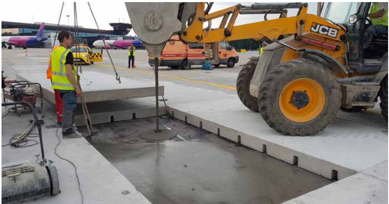
Fig. 6. Installation of a prefabricated concrete slab
