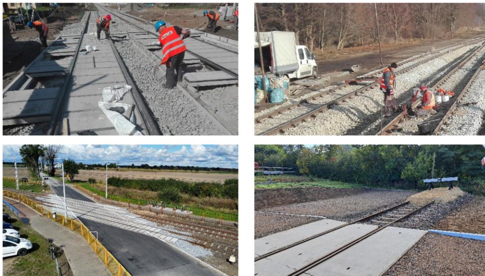
Fig. 2. Examples of the implementation of maintenance and construction work (Portfolio of Remtor sp. z o.o., 2023)
