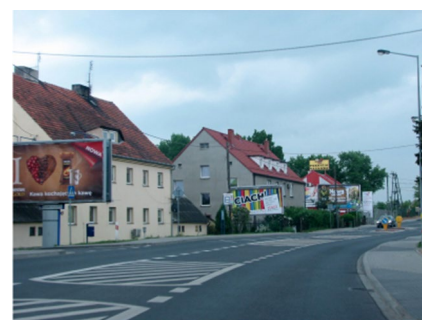
d) The components that make up the structure of the road way
