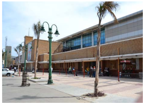
Fig. 6. The new facade with new finishing materials over the old train station building causing aesthetic pollution
