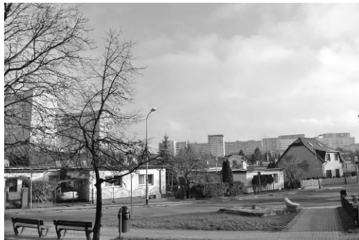
Fig. 29. Houses at Jodłowa Street. Single and multi-family houses. Source: author
