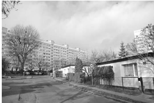
Fig. 27. Houses at Jodłowa Street. Single and multi-family houses. Source: author
