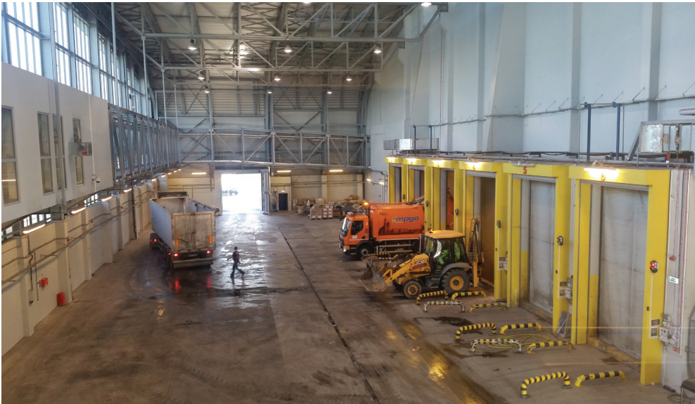
Fig. 3. Unloading of waste to the bunker
