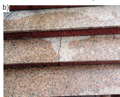
Photo 11. Damage to the cladding of the church entrance stairs: a) loss and damage to the stone and joints; b) cracks of the stone
