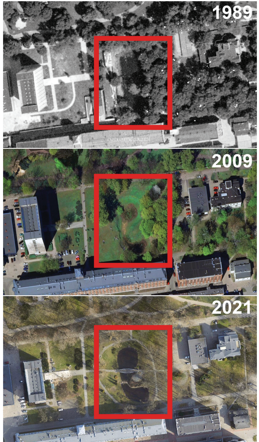
Fig. 2. Aerial pictures showing the reservoir and its surroundings in the years 1989 (reservoir still in its original shape), 2009 (nearly dried-out reservoir), 2021 (current state after regeneration); source: Łódzki Internetowy System Informacji Przestrzennej
