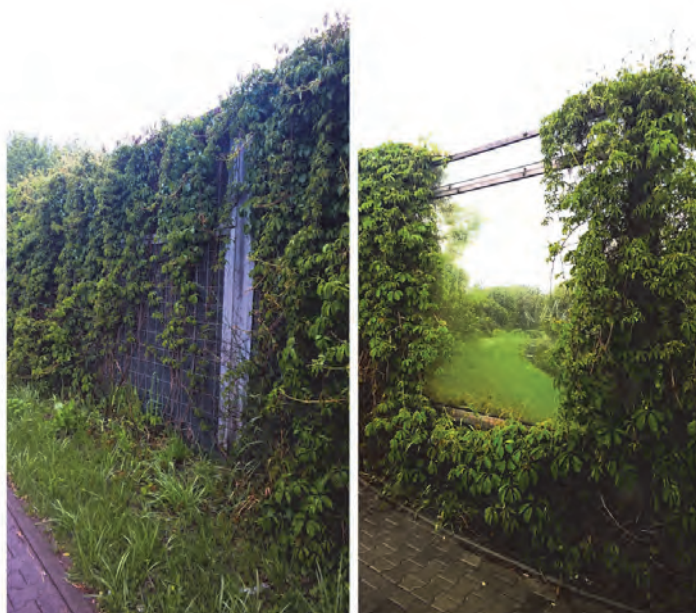
Phot. 1. The noise barrier in the research area "A": "green wall" and transparent acrylic glass panels (photo M. Jakubiak)
