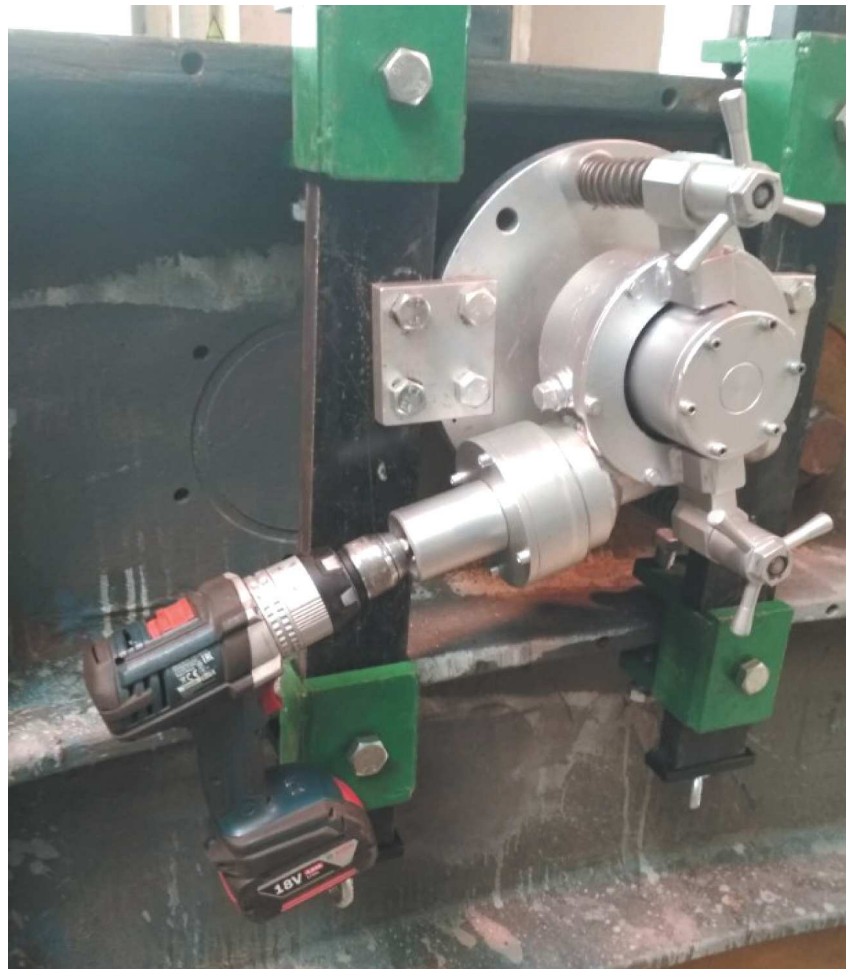
Fig. 10. Milling machine mounted to tubing lining with drill-driver driving the system
