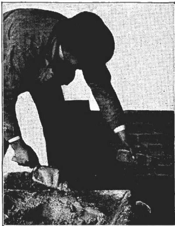
Fig. 1. From the book Bricklaying system , chapter: Training Apprentices, Picking up stock with both hands at the same time; source: Frank B. Gillbreth (1911), Bricklaying system .
