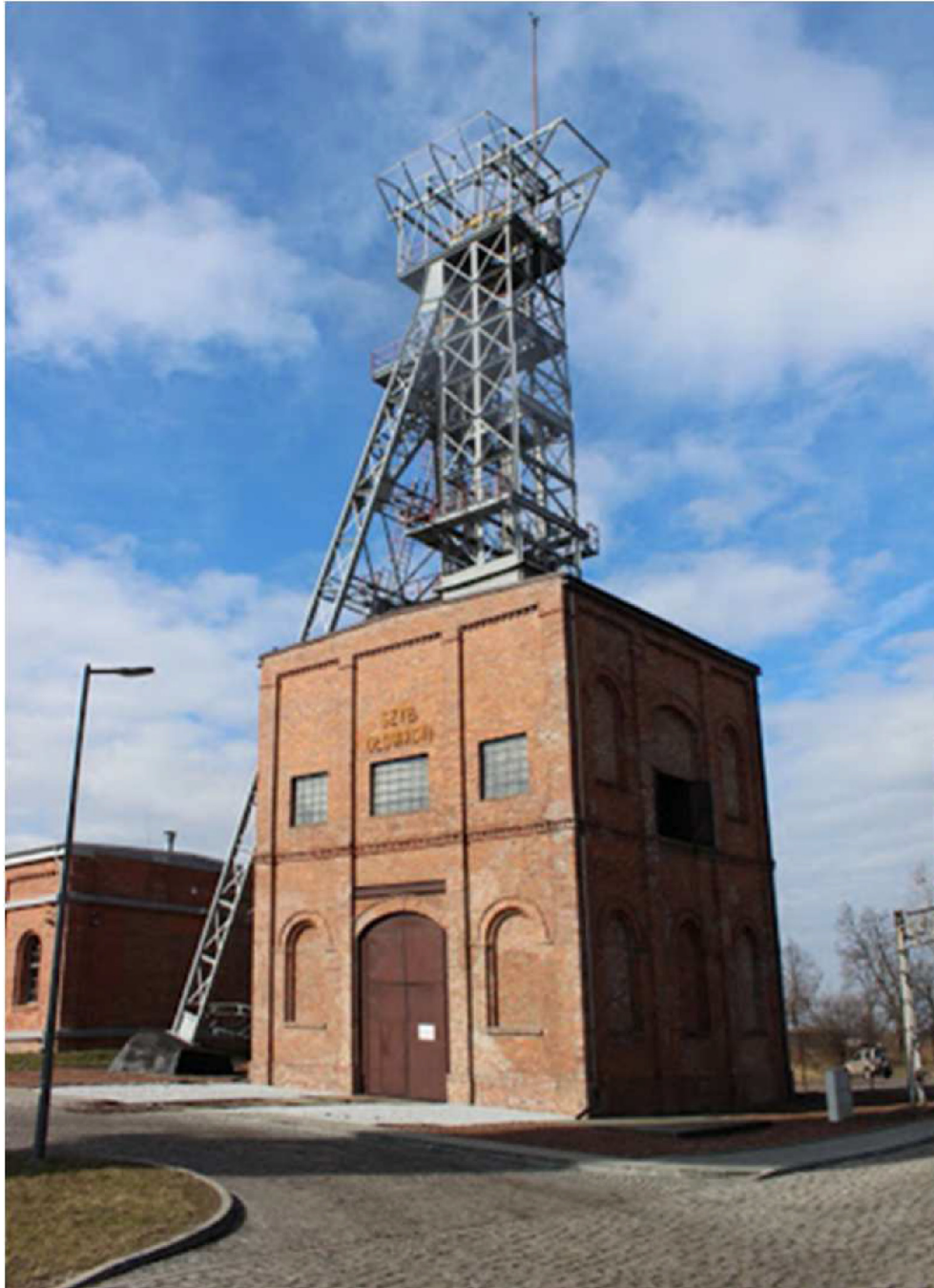
Fig. 2. Glowacki shaft tower.
