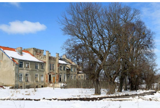
Fig. 10. Present condition of garden palace complex in Stachowizna (photo by K. Ruszczycka, 2013)
