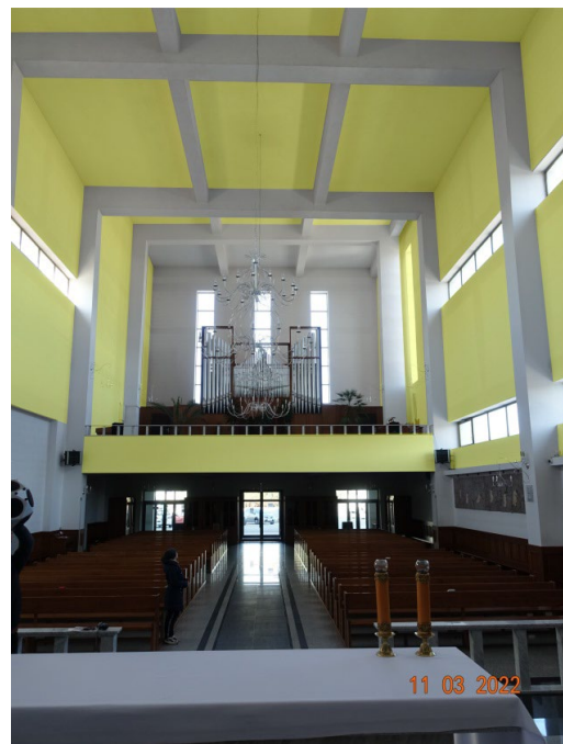
Figure 10. Choir, parts of the ceiling and side walls.
