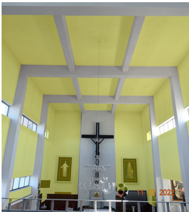
Figure 9. Presbytery, parts of the ceiling and side walls.
