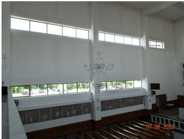
Figure 4. Left wall of the nave.
