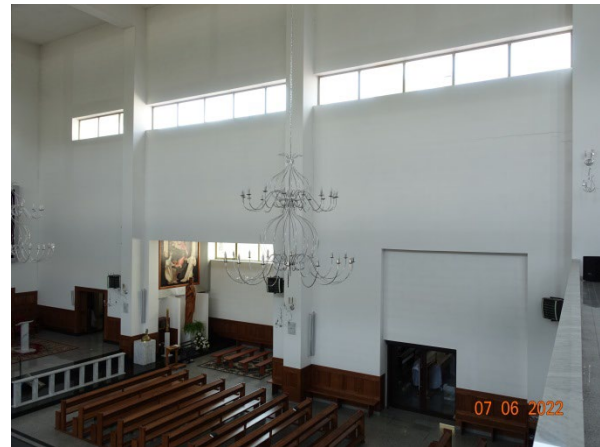
Figure 5. Right wall of the nave with a small nave.
