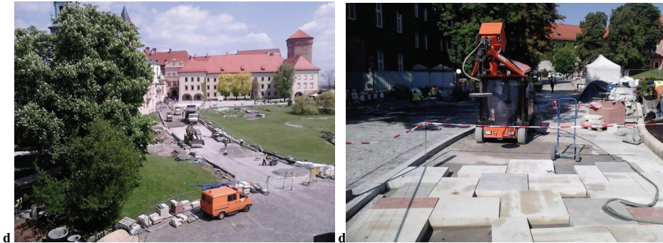
Fig. 1. Fragment of the photographic documentation of refurbishment work performed on the Outer Courtyard at Wawel Castle: (a) view of the bottom of the excavation trench; (b) uncovering of archaeological artefacts; (c) view of the aggregate subbase course being laid; (d) wearing course out of sandstone tiles, source: original photographic documentation.
