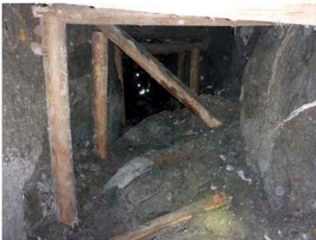
Figure 13. Collapses in the underground gallery caused by damage occurred to the timber support
