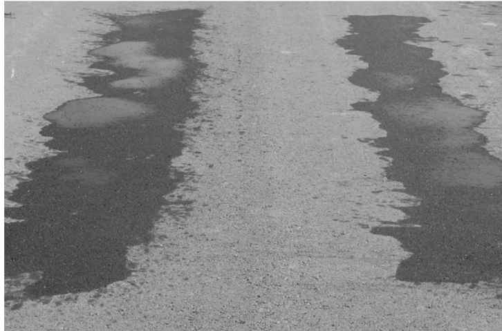
Fig. 1. View of the asphalt roadway dry polluted with diesel [4]
