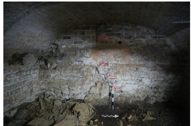
Fig. 7. Visible in the crypt under the north transept is the central north buttress of the body to which the transept wall was added with the first half of the 13 th century levelling layer present beneath them, the lowest parts of the foundations are missing (elaborated by R. Biel)
