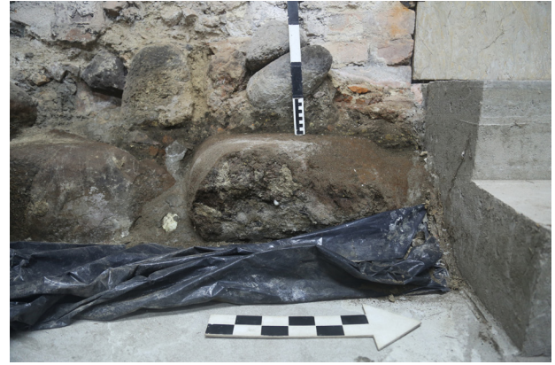
Fig. 6. Clearly visible layer of humus separating the lowest part of the foundations from the proper walls of St Matthias Church (photo by R. Biel)
