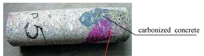
Fig. 17. Drilled core with carbonized concrete marked using rainbow test (Ref. 56)
