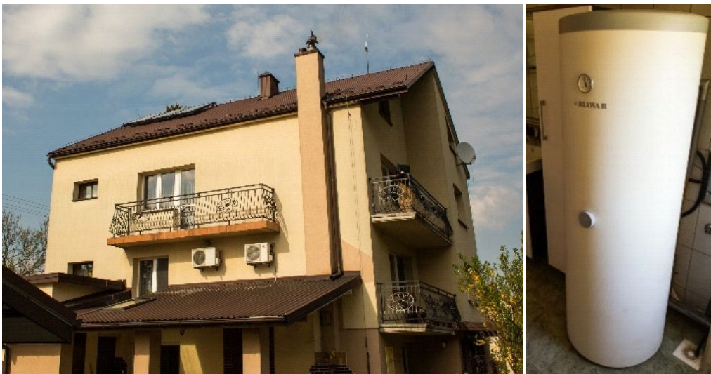
Fig. 1. The detached house and the solar storage tank inside Source: own study
