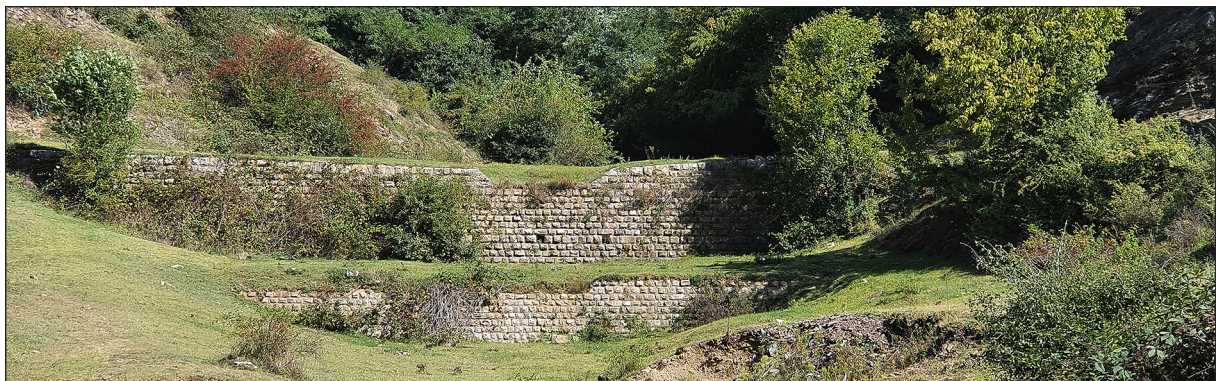
Fig. 10. Soil erosion practice in the basin slopes
