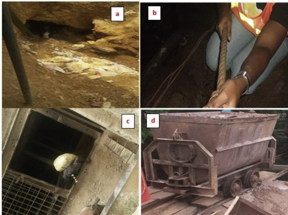
Fig. 4 – (a) Adit, (b) Descending into a stope using rope, (c) Miner carries broken rocks on the back, and (d) Wagon for carrying materials by pushing.
