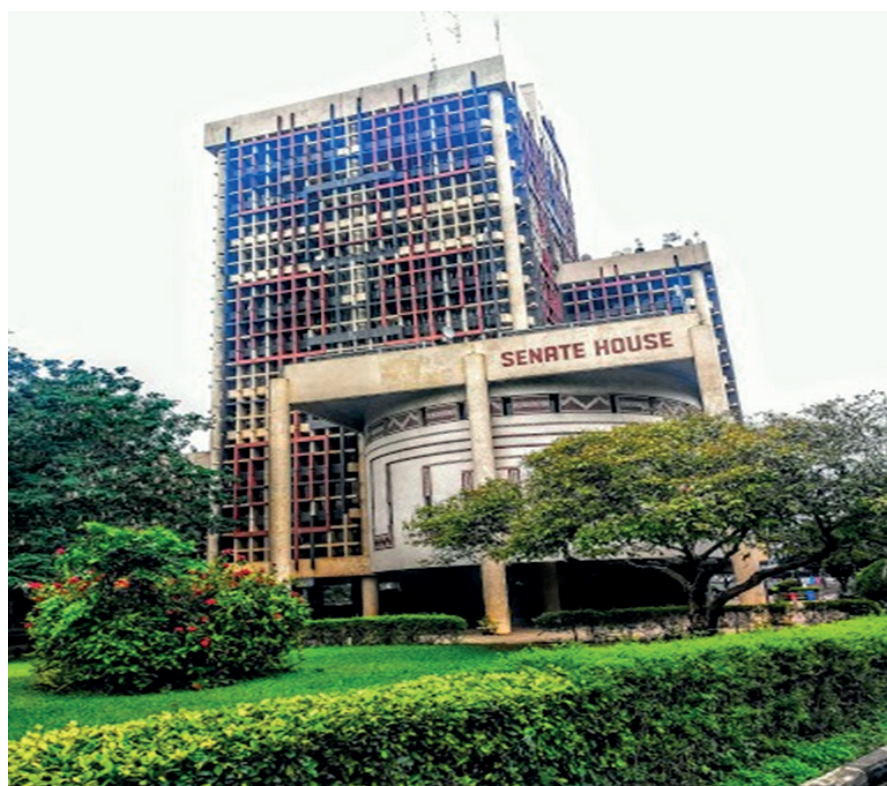
Fig. 1. University office complex
