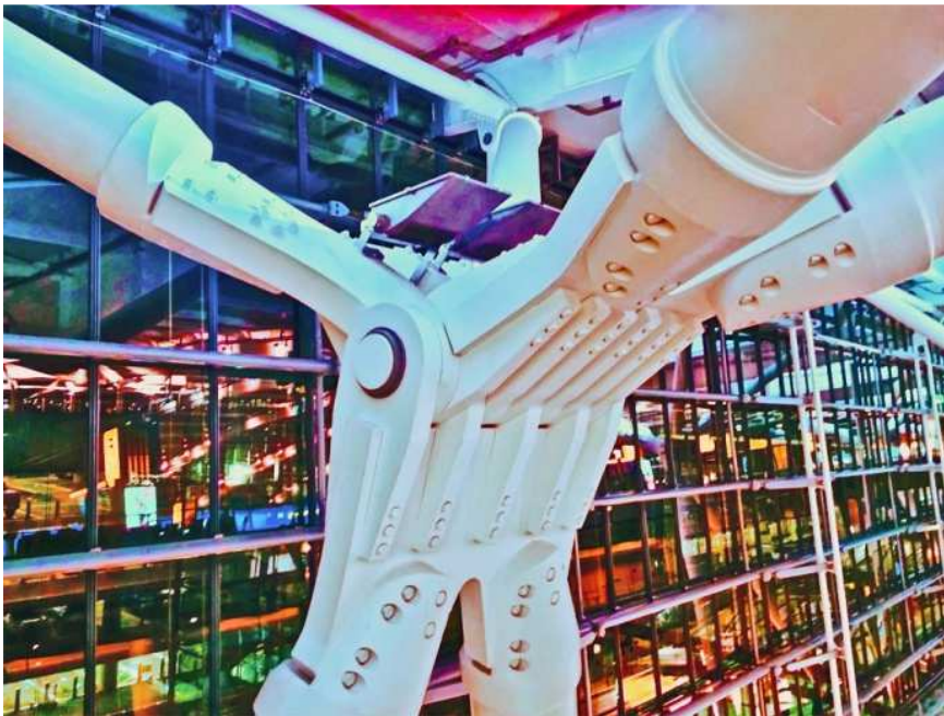
Fig. 10. The joint of steel spatial structure at Heathrow airport, London, England (author of photography: Andreas Komodromos [10])
