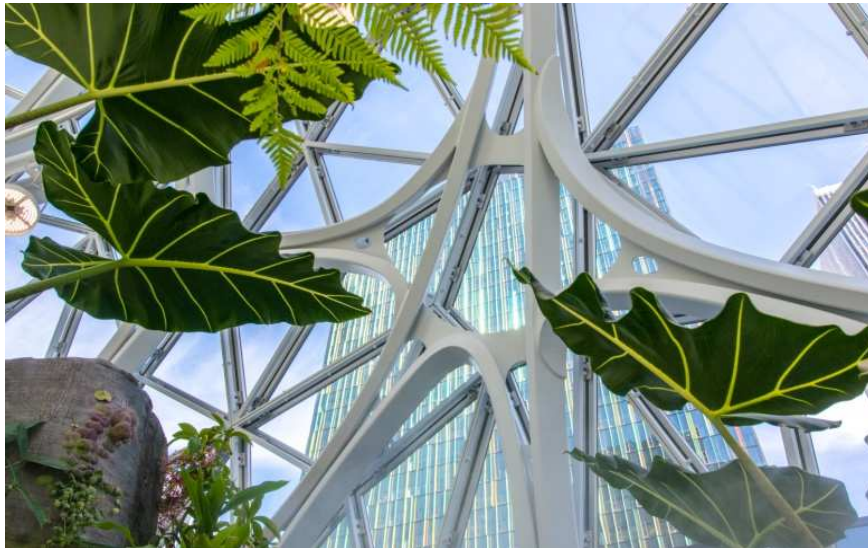
Fig. 7. Amazon Spheres – spherical conservatories serve as employee lounge and workspace located on the headquarters campus of Amazon company in Seattle, USA, completed in January 2018: connections details (author of photography: Manuel Bahamondez H [10])
