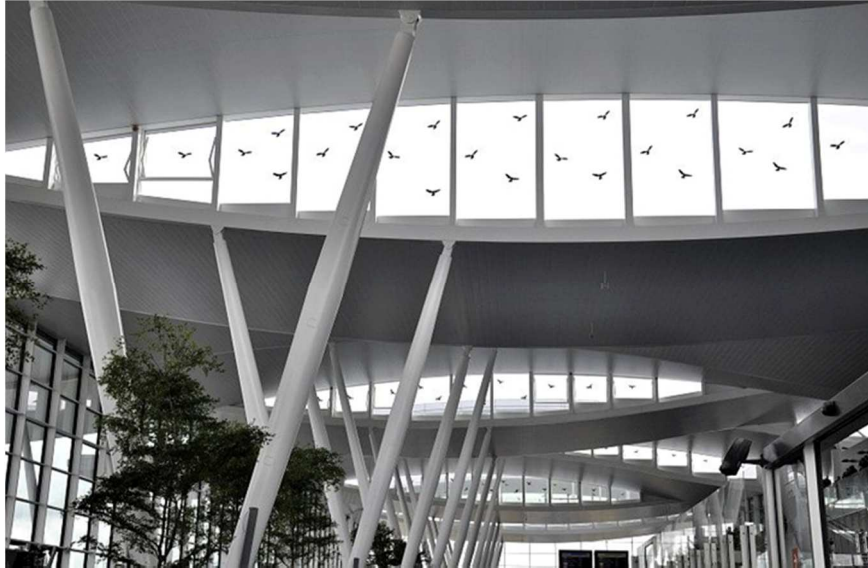
Fig. 5. Copernicus Airport Wrocław, Wrocław, Poland (author of photography: Paweł Żwirek)
