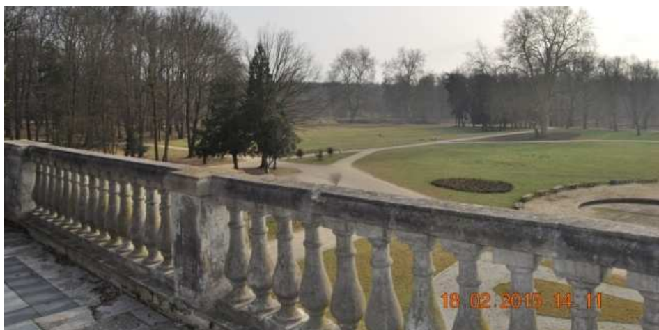
Fig. 8. View of the park following renovation (fot. W. Sokołowski)
