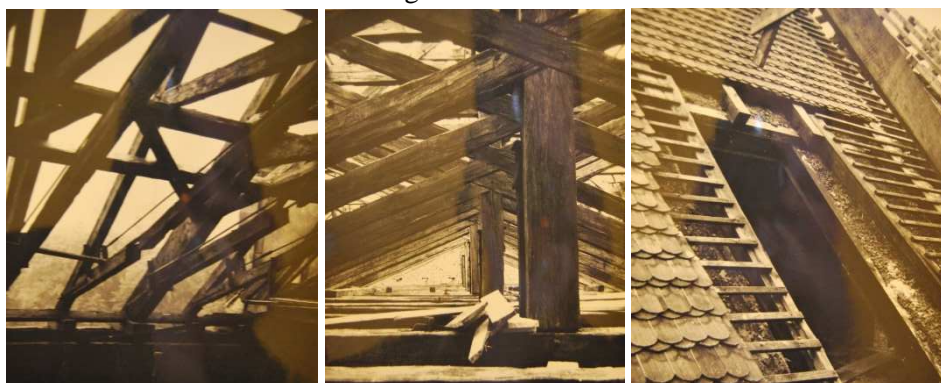
Fig. 5-7. Photographs of the palace roof taken in 1972 (fot. M. Świątek)
