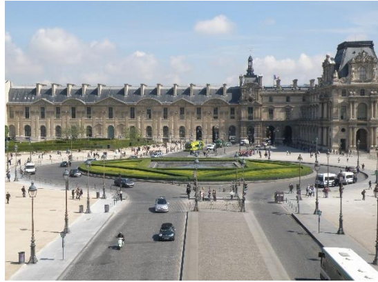
Fig. 6. An interesting arrangement of a central island with the use of low greenery in the roundabout localized near the Louvre Museum in Paris (France)
