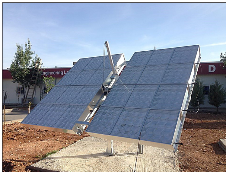
Figure 5. One of the CPV units installed in the site
