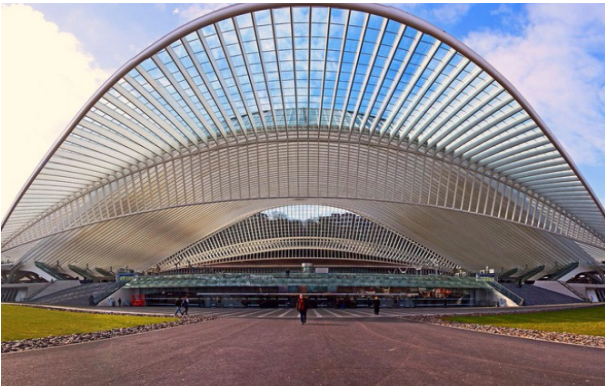
Fig. 6. Liège-Guillemins Railway Station.
