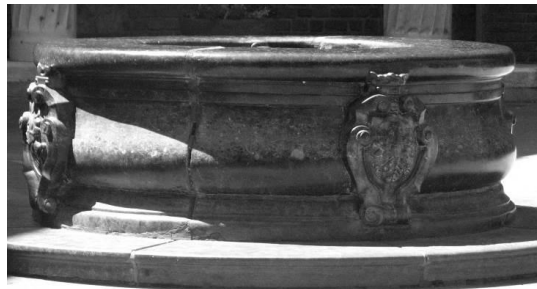
Fig.10 Well in the courtyard of the Collegium Maius made of Dębnik “marble”
