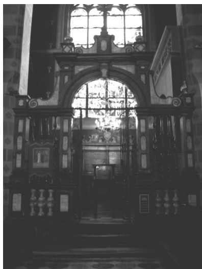
Fig. 12. Side chapel of south nave – St. Lazarus chapel in St. Marys Church – encrustations of Paczółtowice “marble” in Dębnik limestone in gates of chapel
