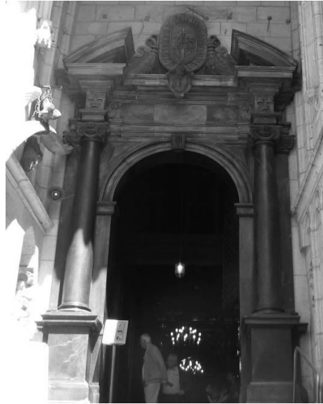
Fig. 9. Portal of main entrance to the Wawel Cathedral made of black Dębnik “marble”.
