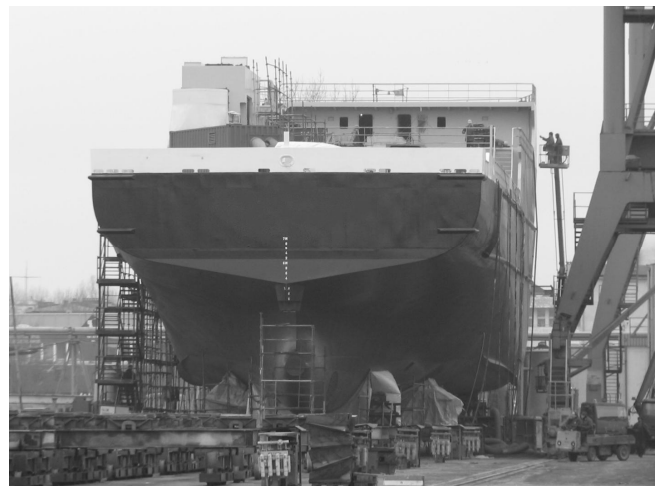
Figure 1. The ship at the repair post R1/B1
