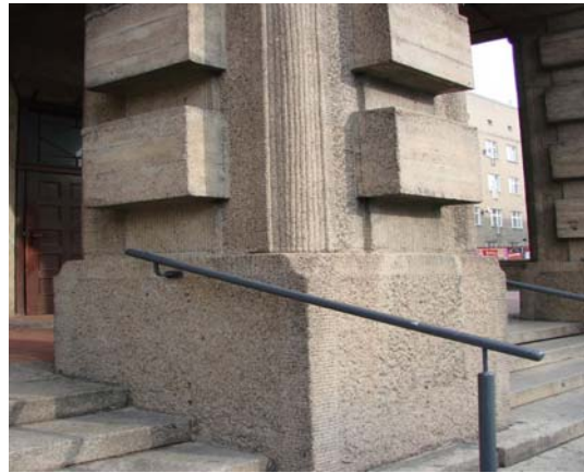
Fig. 1a. Manifestation of the modern, concrete architecture of the Garnisonkirche (1913-1919) in relation to the opposite, neogothic, brick body of the Bugenhagen Church in Szczecin. Source: Halina Rutyna . 1b. Modernist concrete detail: raw base and column supporting the entrance tint with the texture of a roughly corrugated concrete expedition; currently conducted restoration works are being done according to research and design by architect Halina Rutyna - Atelier Architektury i Konserwacji Zabytków. Source: Halina Rutyna
