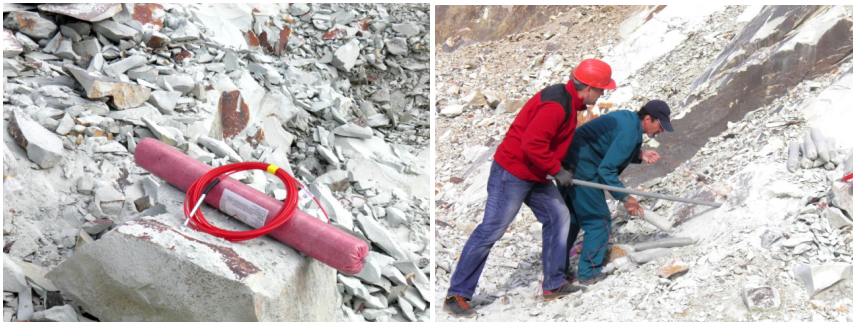
Fig. 6. EURODYN explosives and borehole charge.
