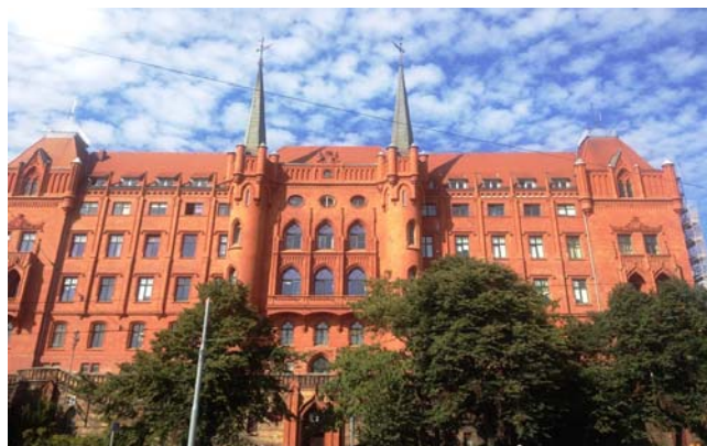
Figure 2. Building housing the RIS-PL Operating Centre. Source: Own work, based on [15].
