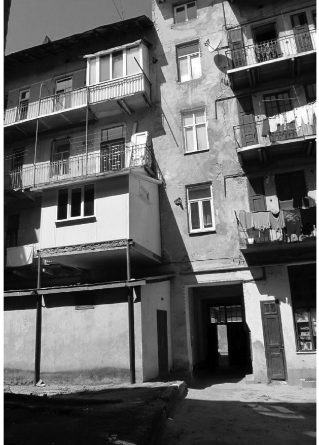
il. 4. Courtyard on 82 Khmelnytskoho Street – example arranging annex to the building at ground and first floors (photo by author)
