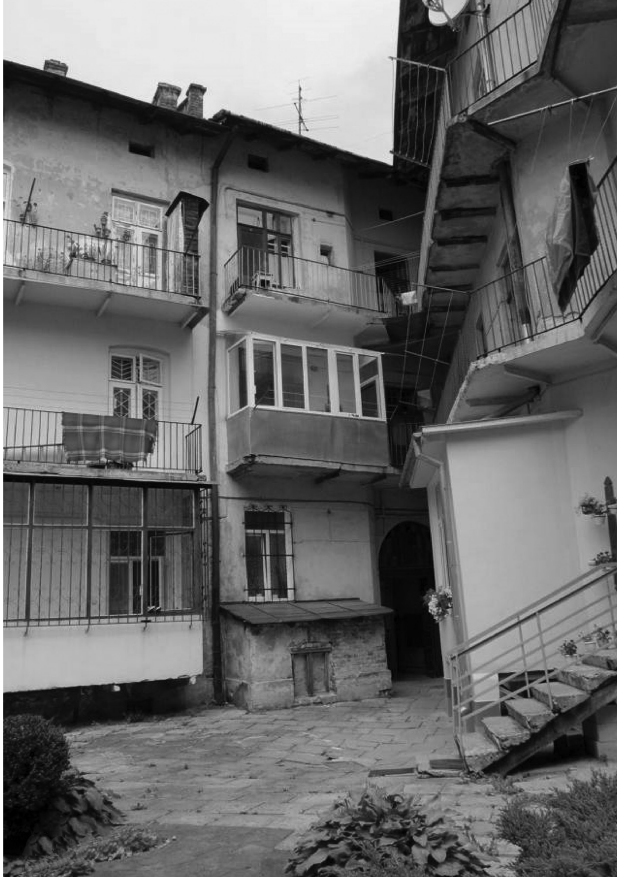
il. 3. Courtyard on 15 Korolenka Street – example arranging annex to the building and galleries glazing (photo by author)
