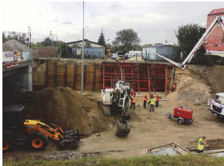
Figure 3. Excavation of existing embankment
