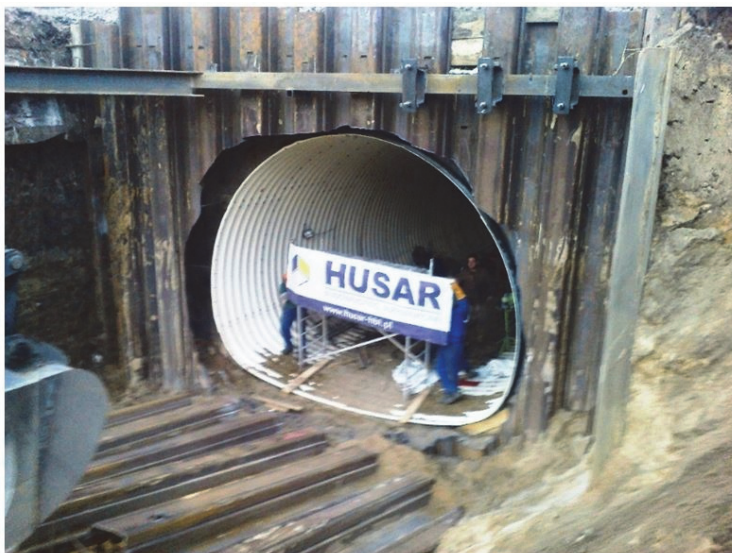
Figure 5. Merge between two phases of construction
