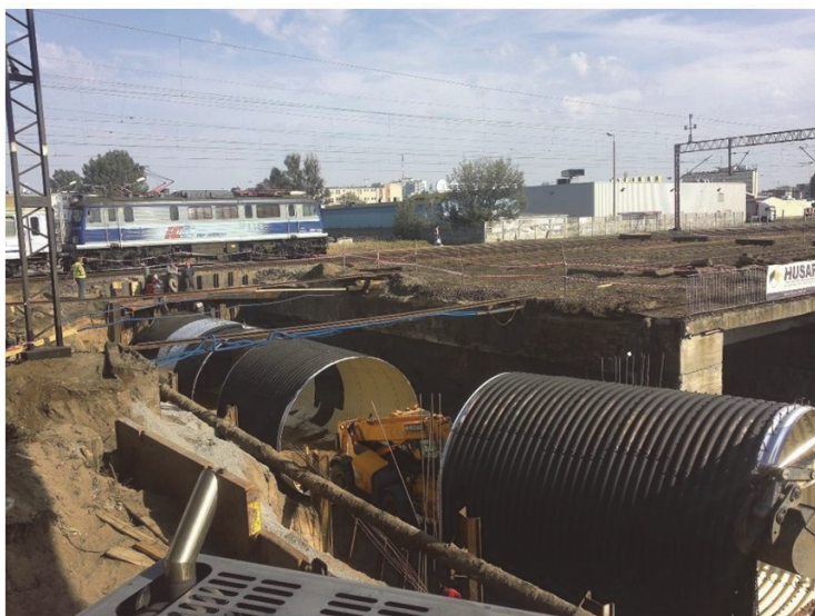
Figure 4. Assembly of steel structure
