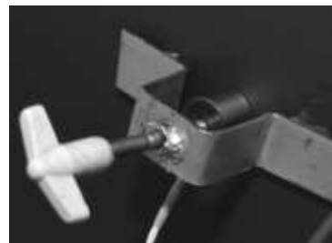
Fig. 4. Piezoelectric AE transducer WD AH17 installed on the tank wall
