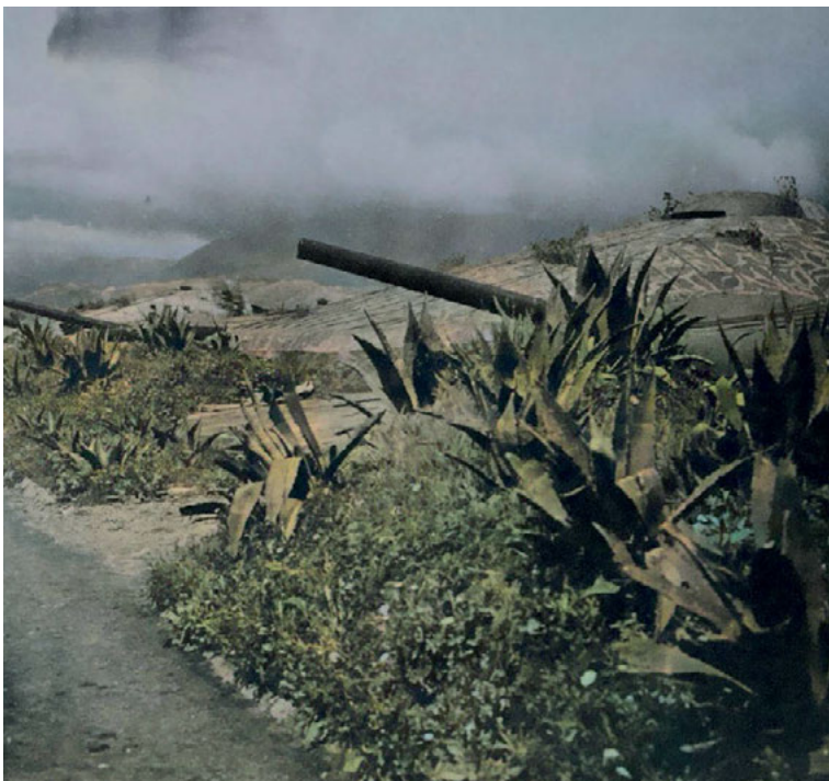
Ill. 9. Archival photograph of Caballa coastal battery (Kotor, Montenegro), colorized. Well-visible combination of two-tone camouflage painting, live vegetation found locally, and supplemental masking with cut branches around the observations post's armored cupola. Authors' own work based on original photo, Österreichisches Staatsarchiv — Kriegsarchiv, Wien, file ref. AT-OeStA/KA BS I WK Fronten Serbien, 2499.
