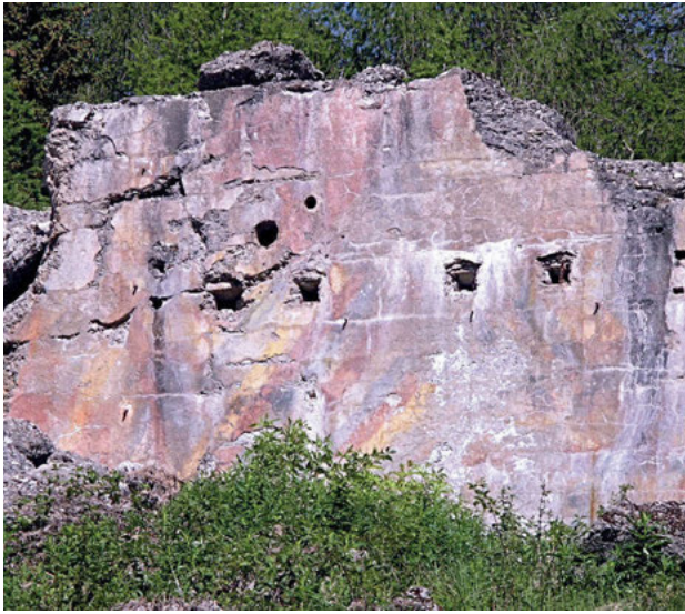
Ill. 7. Fort Tonale, present condition (2018). Preserved relics of camouflage paint on the ruins of the fort's concrete barracks. A layer of rubble shielded it from weathering. Larger patches of deforming mask (ca 1–2 m 2 size) were composed of small mimetic patches (about 20 cm wide). Photo by the authors.
