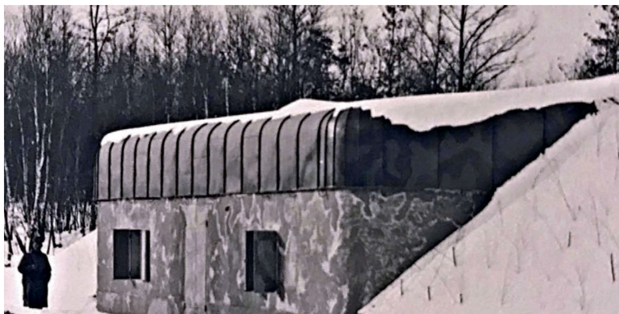
III. 2. Wolski Las ammunition shelter in Kraków, Poland, c. 1915. The building was erected during the 1914–1915 construction season and covered with tricolour camouflage. Print of the photograph is in the authors' private collection.
