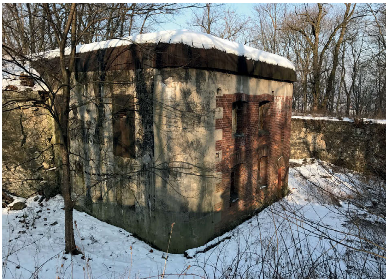
Ill. 4. Fort Winnica in Kraków, Poland, current status (2020). The fort was built between 1898–1899. Visible relics of the tar spots of the primer camouflage layer. Photo by the authors.
