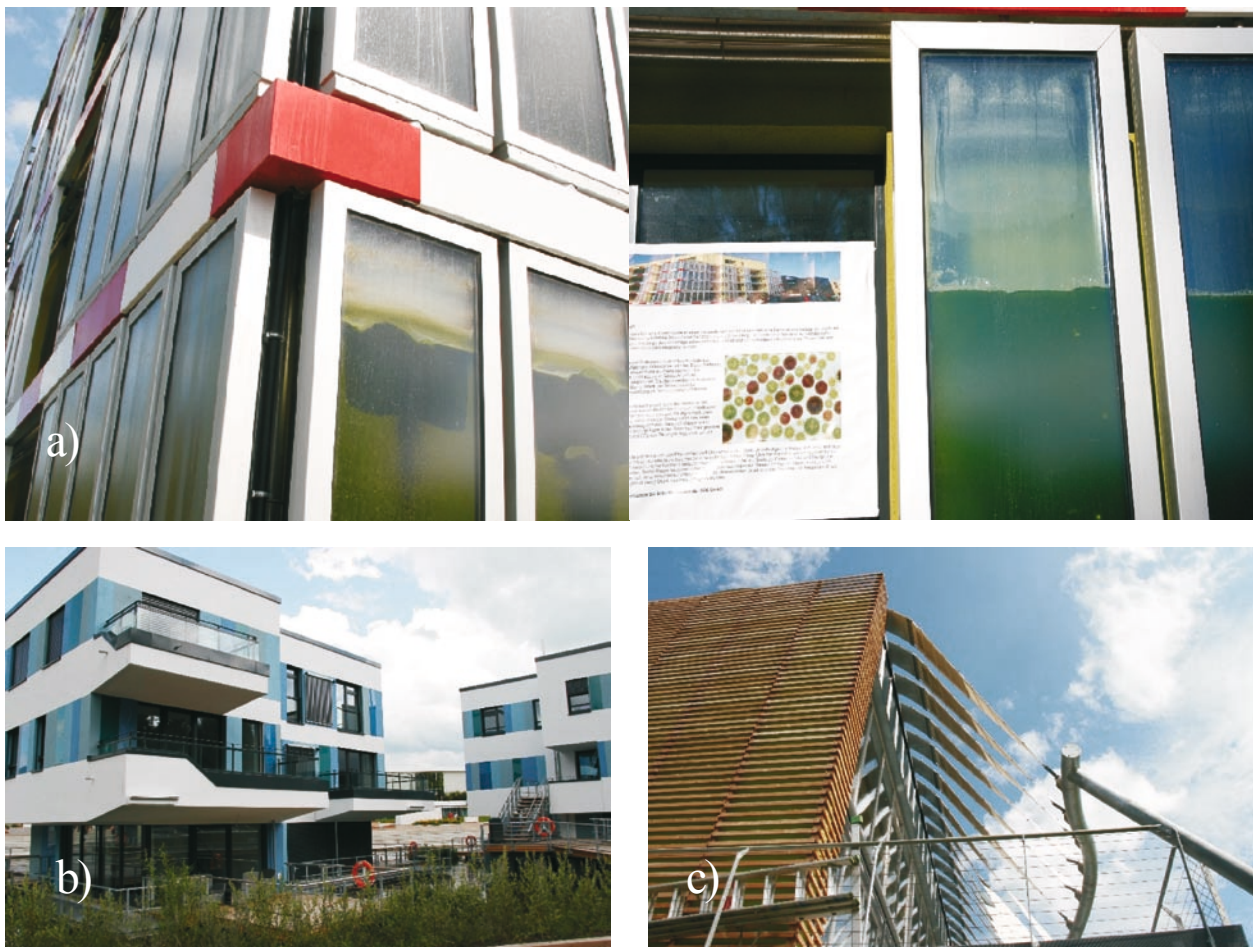
Fig.4 a Hamburg - BIQ building and section of algal bioreactor, design. Splitterwerk, 4.b. WaterHouses, design. Schenk + Waiblinger, 4 c. SOFT HOUSE building ,design. Kennedy & Violich, Architecture source: photo by the author
