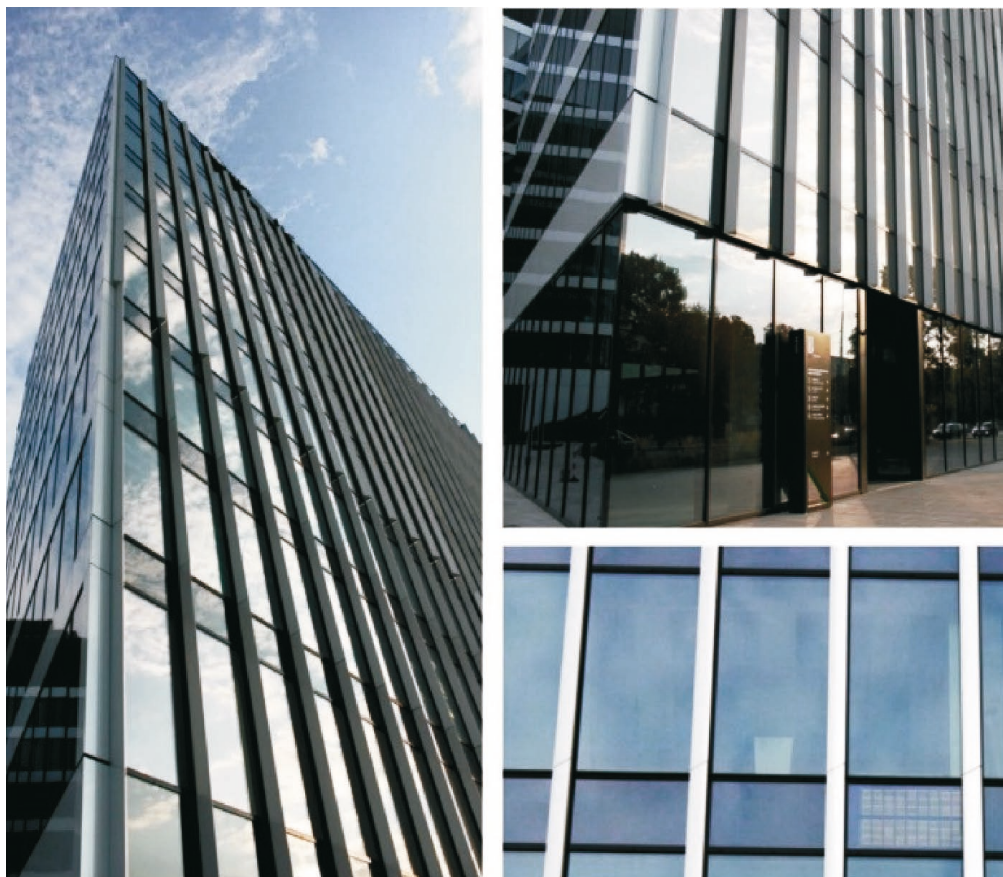
Fig. 5a. Warsaw, office building Spark C, Skanska – Warszawa 2018 and ultra-thin perovskite-based photovoltaic cells on the façade. The size of the cell under test is 1.3 x 0.9 m,
