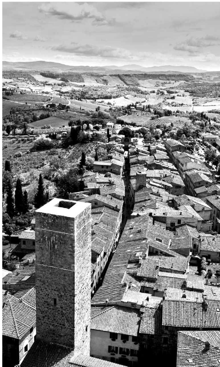
Fig. 2. A comparison between roofscapes of Białystok (Poland; photo by Sara Doriguzzi Zordanin) and San Gimignano (Italy, photo by Alex Da Canal) showing the difference in scale, forms and materials
