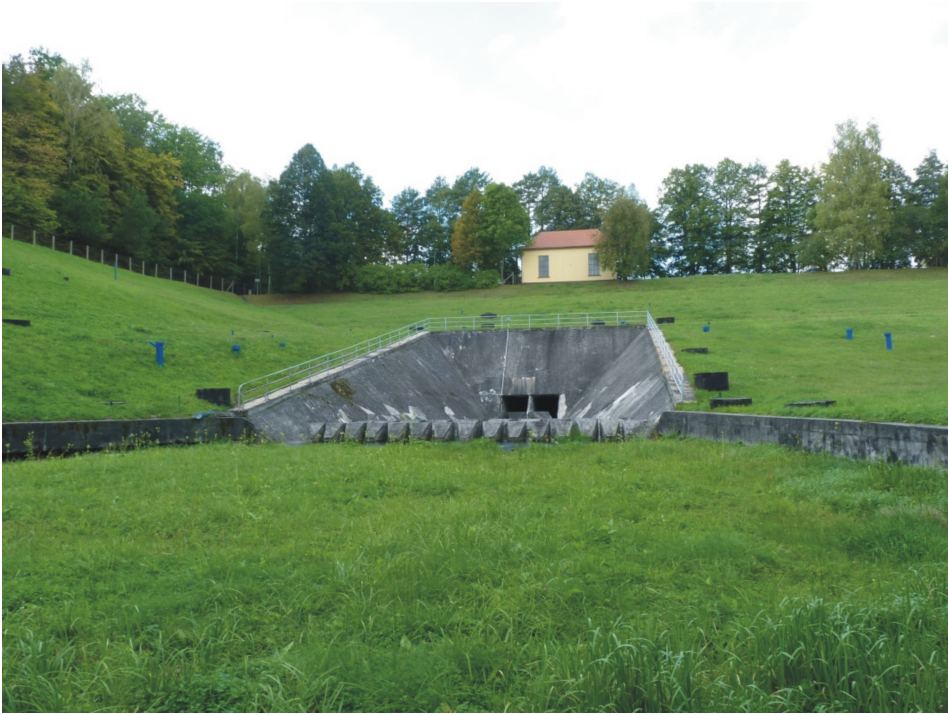
Fig. 1. General view of the Zur earth dam and the bottom outlet
