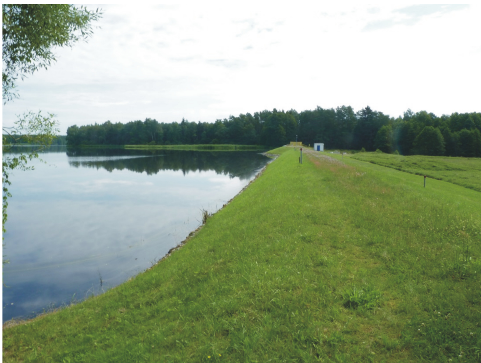
Fig. 2. General view of the Podgaje earth dam
