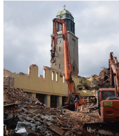
Fig. 4. Demolition of the Church of St. Joseph – 2016
