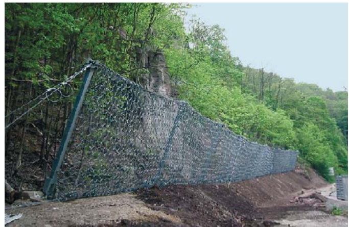
Fig. 7. Installed RX-300 Rockfall Barrier with a designed absorption capacity of 3,000 kJ
